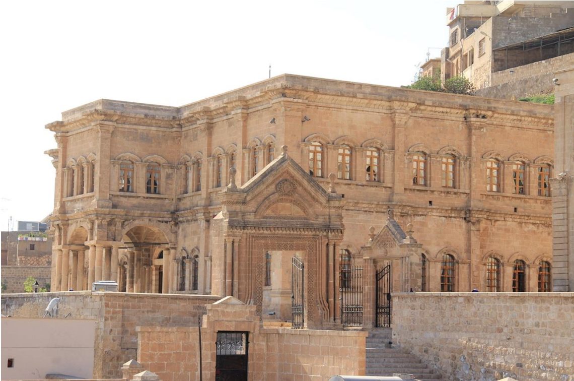
Figure 10. Rüşdiyye School. General view.
