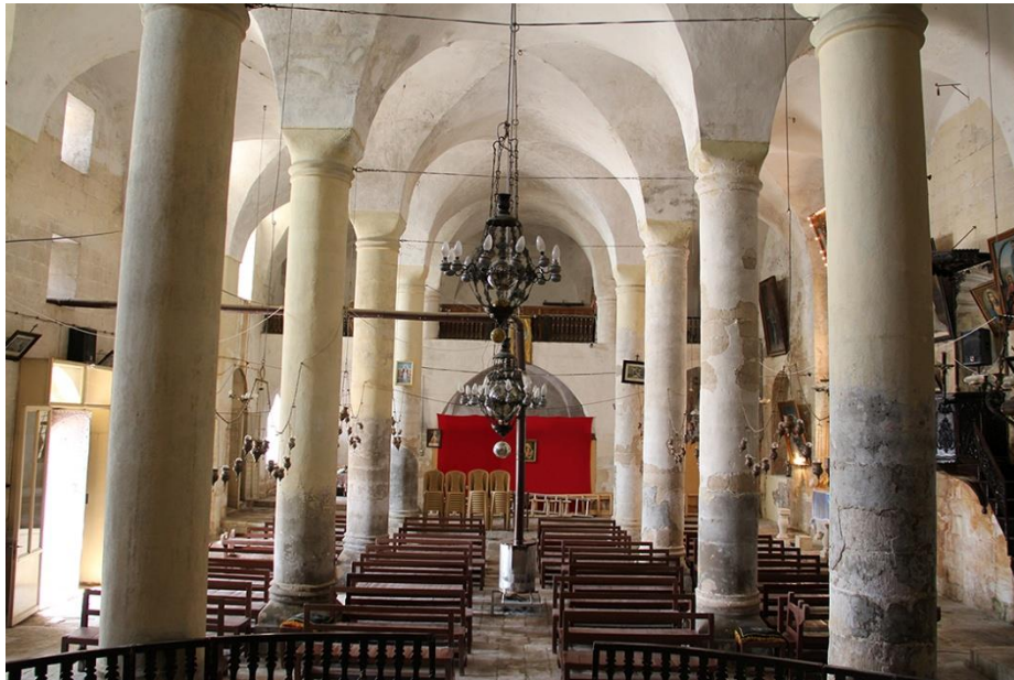
Figure 15. Virgin Mary Church. Interior. Columns supporting cross vaults.
