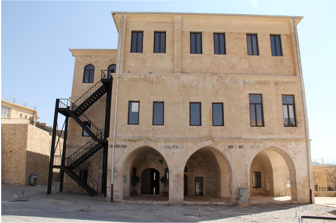
Figure 7. Government Palace. View of west façade.
