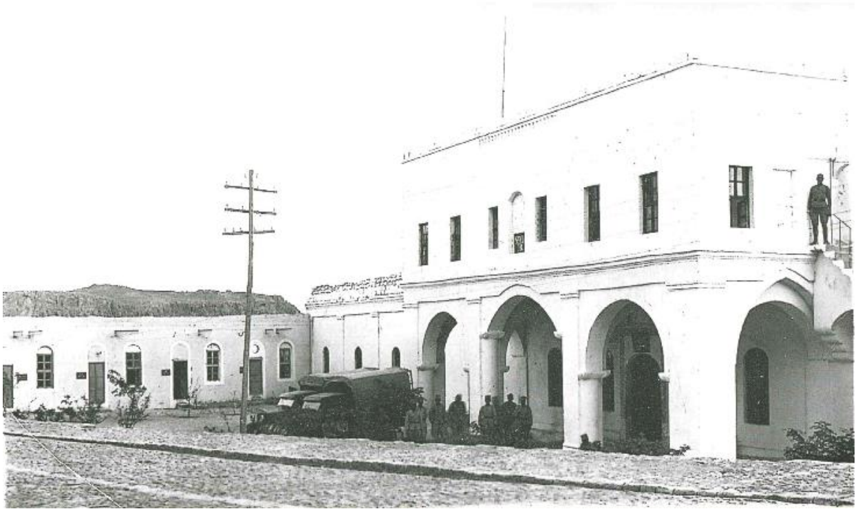
Figure 6. View of Revenue Hall and Military Barracks (Bekin 2010: 167).
