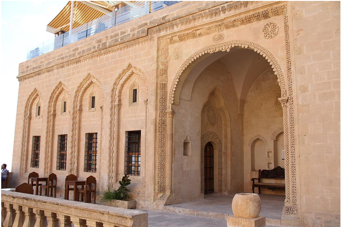
Figure 18. Şahtana House. Southern façade and iwan.
