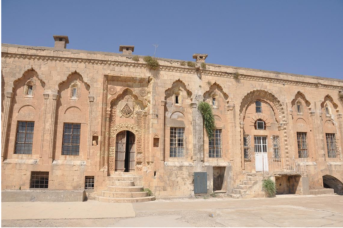
Figure 17. Dokmak Family House. General view of the south façade.
